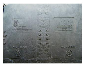
Plate 1: Front view of tile showing manufacturer's details. Note fixing locations.
